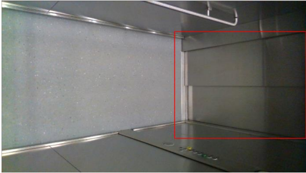
Figure 34 Template matching door closed
